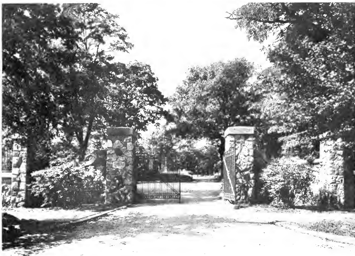
ENTRANCE KENOSHA CEMETERY ASSOCIATION, KENOSHA, WIS. N. MAX DUNNING, ARCHITECT
